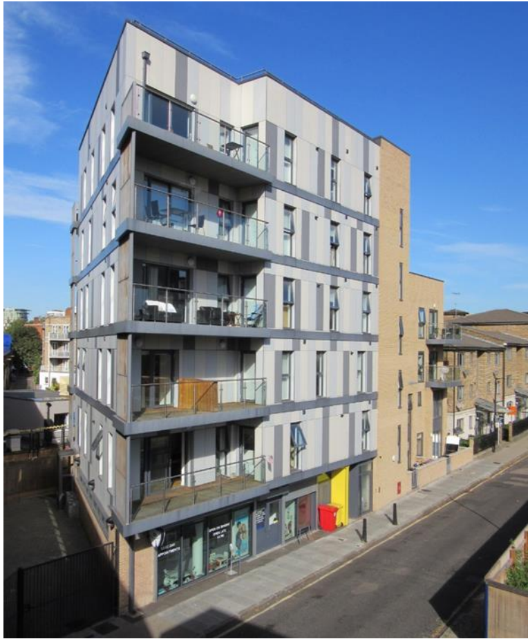
Figure 23 - Cayman Court, taken from Westferry DLR station
