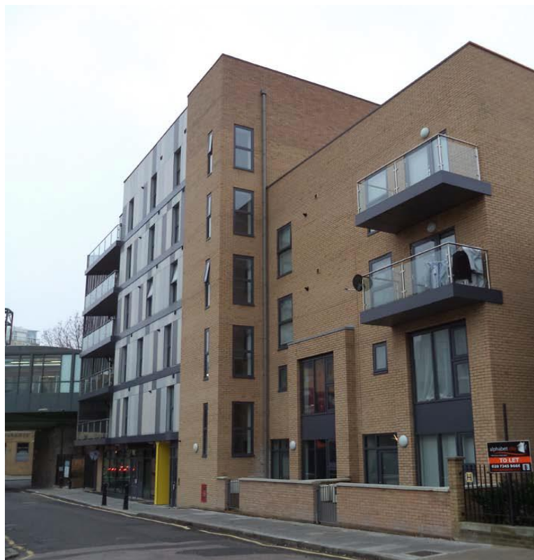
Figure 24 – Cayman Court from Salter Street
